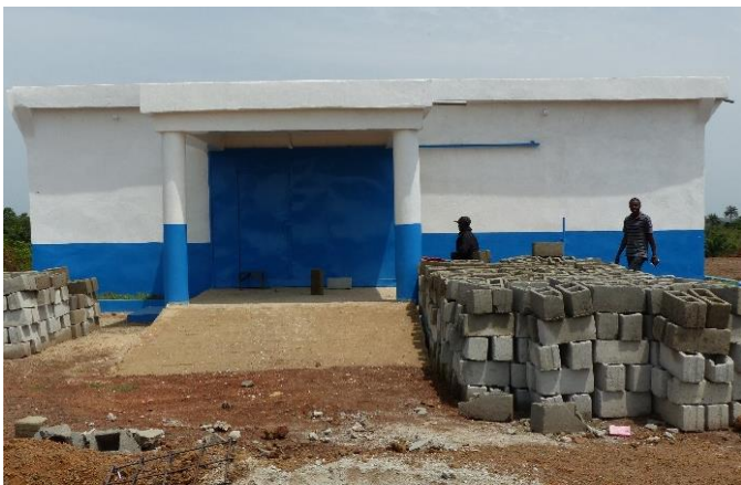
CHAL drug depot in Gbarnga under construction
